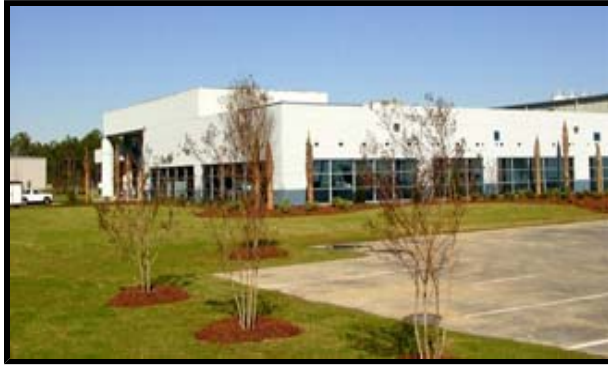
Corning Cable Systems, Inc. Distribution & Manufacturing Facility
