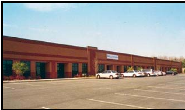
Miller Road Project Office/Warehouse Facilities
