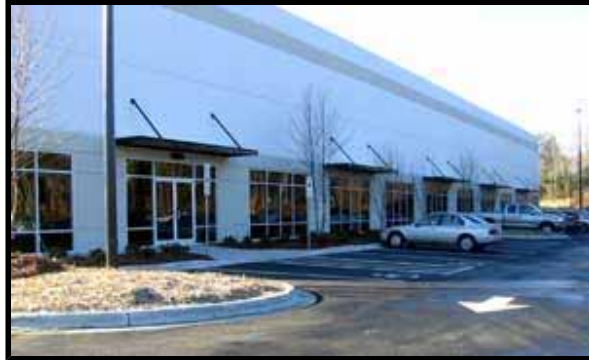
Bonitz Building Concord, NC
