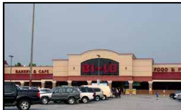
Gateway Village Shopping Center Travelers Rest, SC
