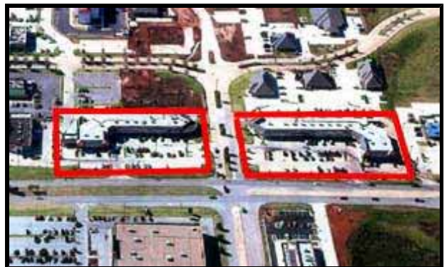
Shoppes at NorthPointe Oklahoma City, OK
