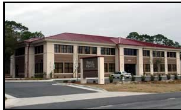
Brock & Scott Office Building
