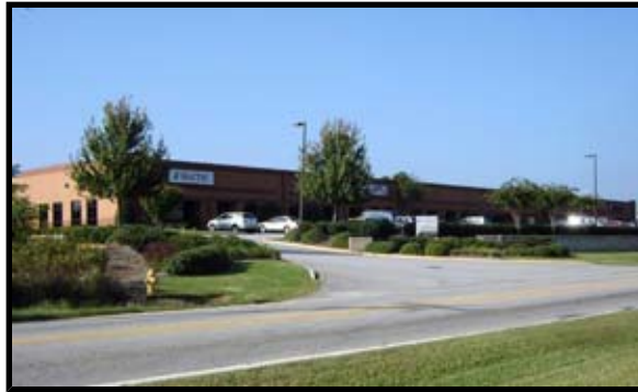
Miller Road Office Building
