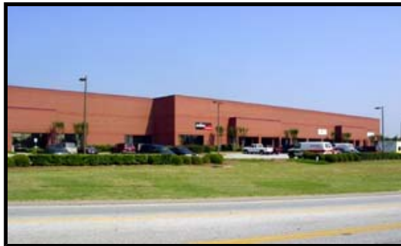
Forrester Park Industrial Building
