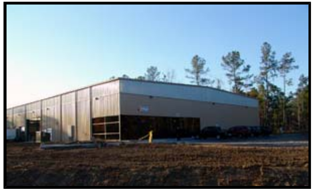
Southern Staircase Summerville, SC
